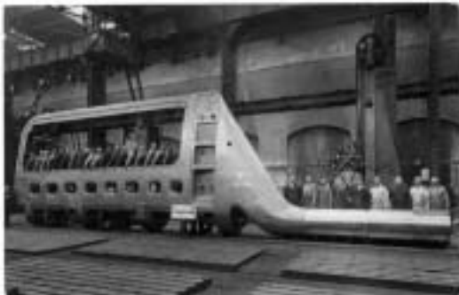
Casting of the rudder frame for the French passenger ship Normandie (1933)
